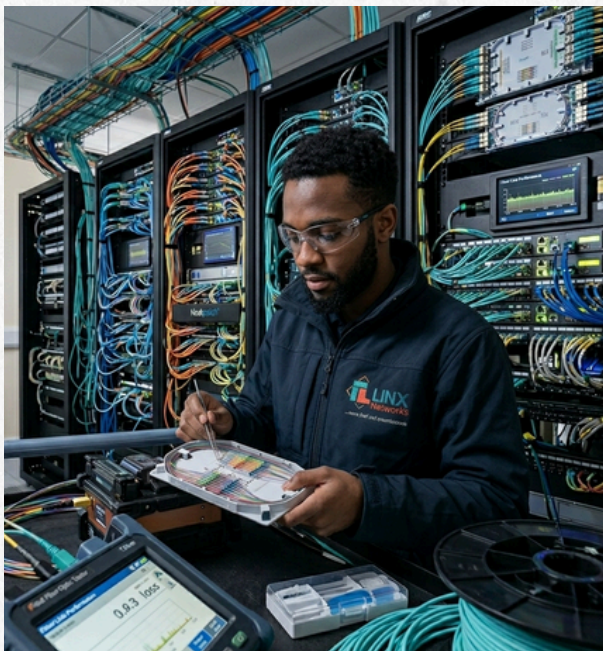
Fiber Optics Splicing and installation Project
